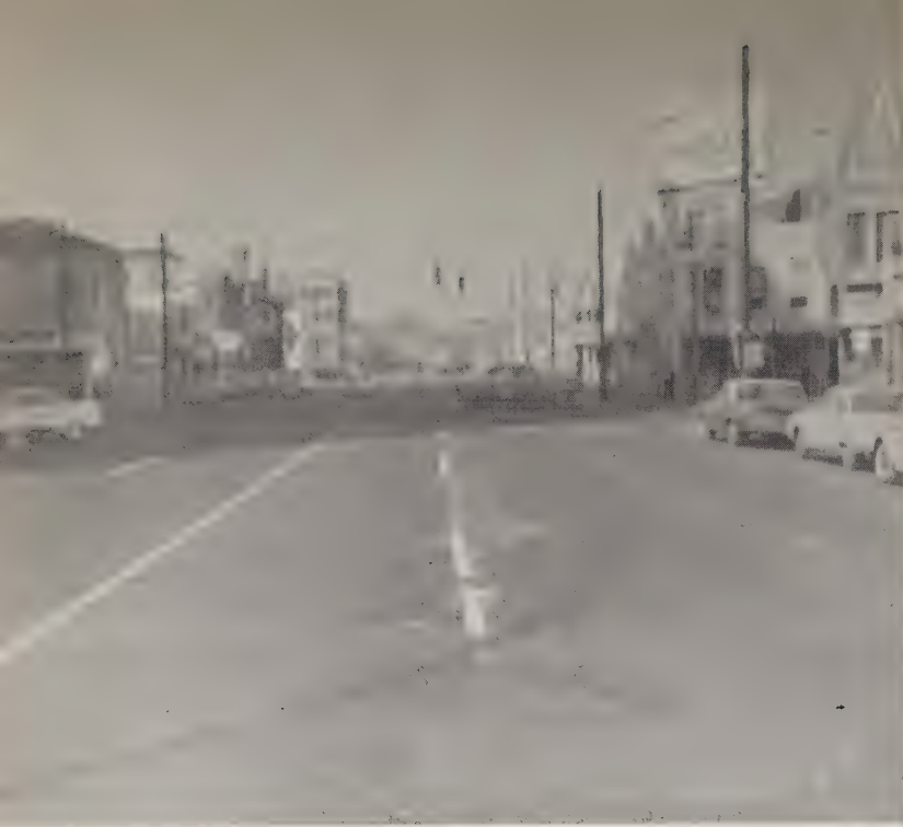
Lee Street looking past the intersection of Montgomery Street towards the depot in 1962. (left)
